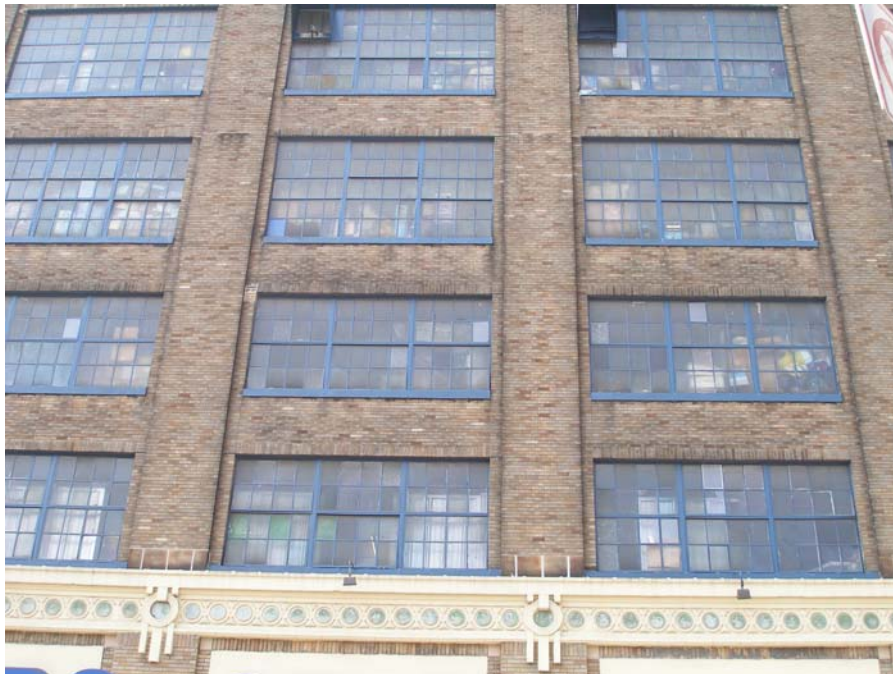
Wheatsworth Bakery Building, 444 East 10 th Street (a/k/a 436-446 East 10 th Street), Manhattan. Photo by Donald G. Presa, June 2008
