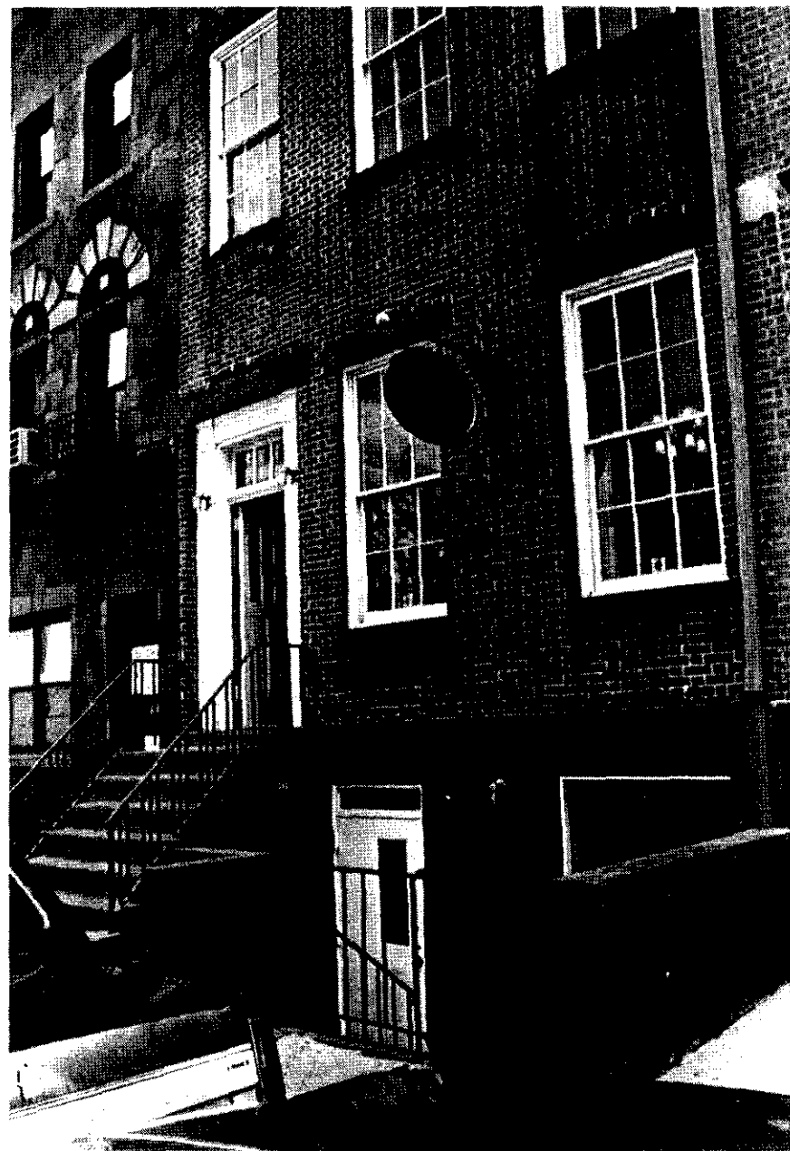
Basement and first story details Photo by: Carl Forster, 1998
