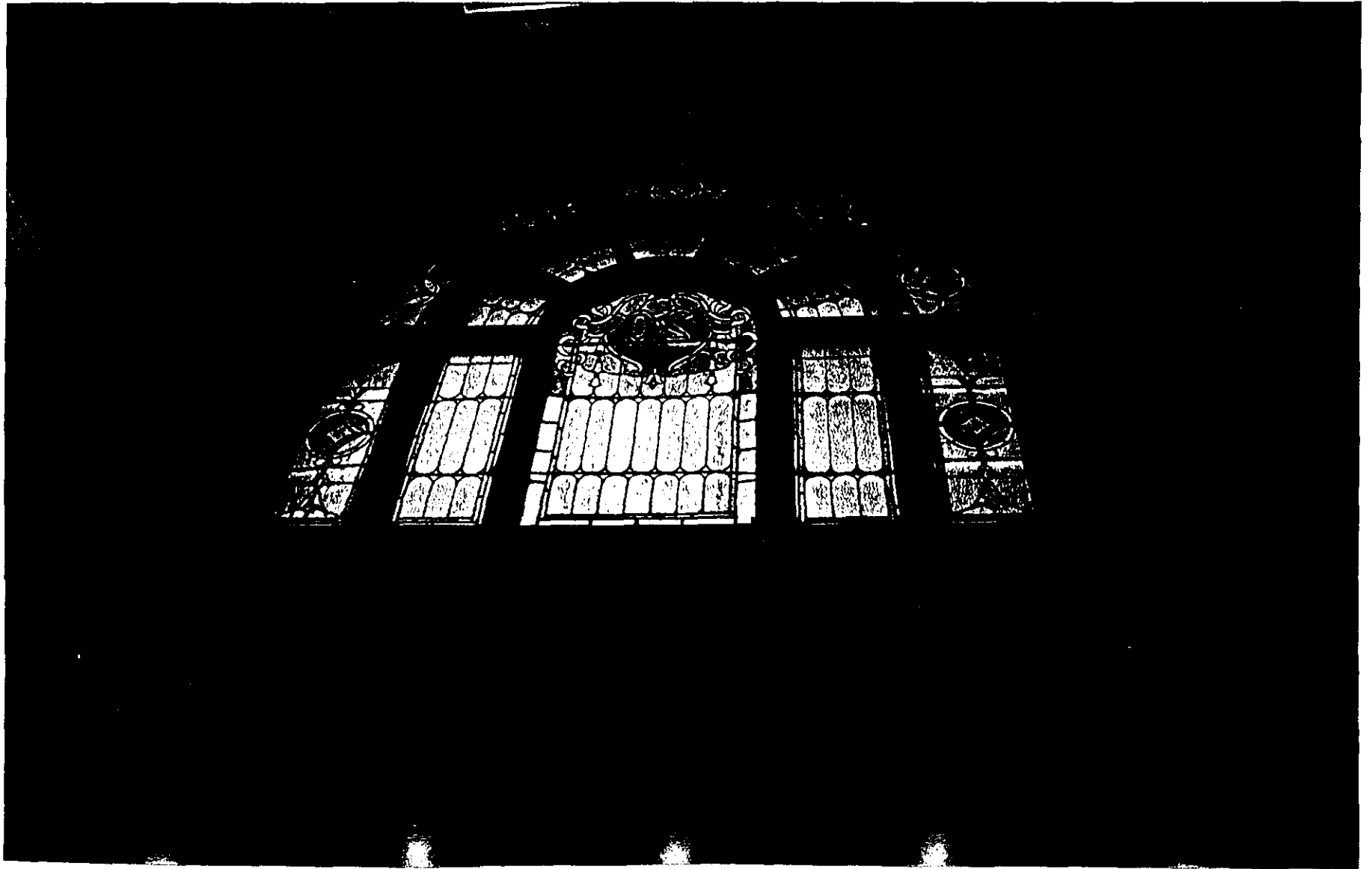
Mechanics' and Tradesmen's Institute Facade, stained glass transom over entrance
